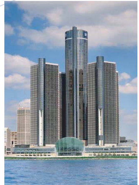
General Motors Global Headquarters at the Renaissance Center - view of the new Winter Garden and waterfront park from the Detroit River, Michigan Photo by GM Worldwide Facilities Group, 2003
