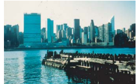
Deteriorating pier on the East River, New York, NY looking towards the United Nations complex Photo by Bonnie Harken, 1991
