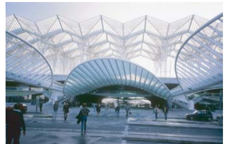
Intermodal connections between rail, bus and metro at the Oriente Station, Lisbon, Portugal Photo by Bonnie Harken, 1998
